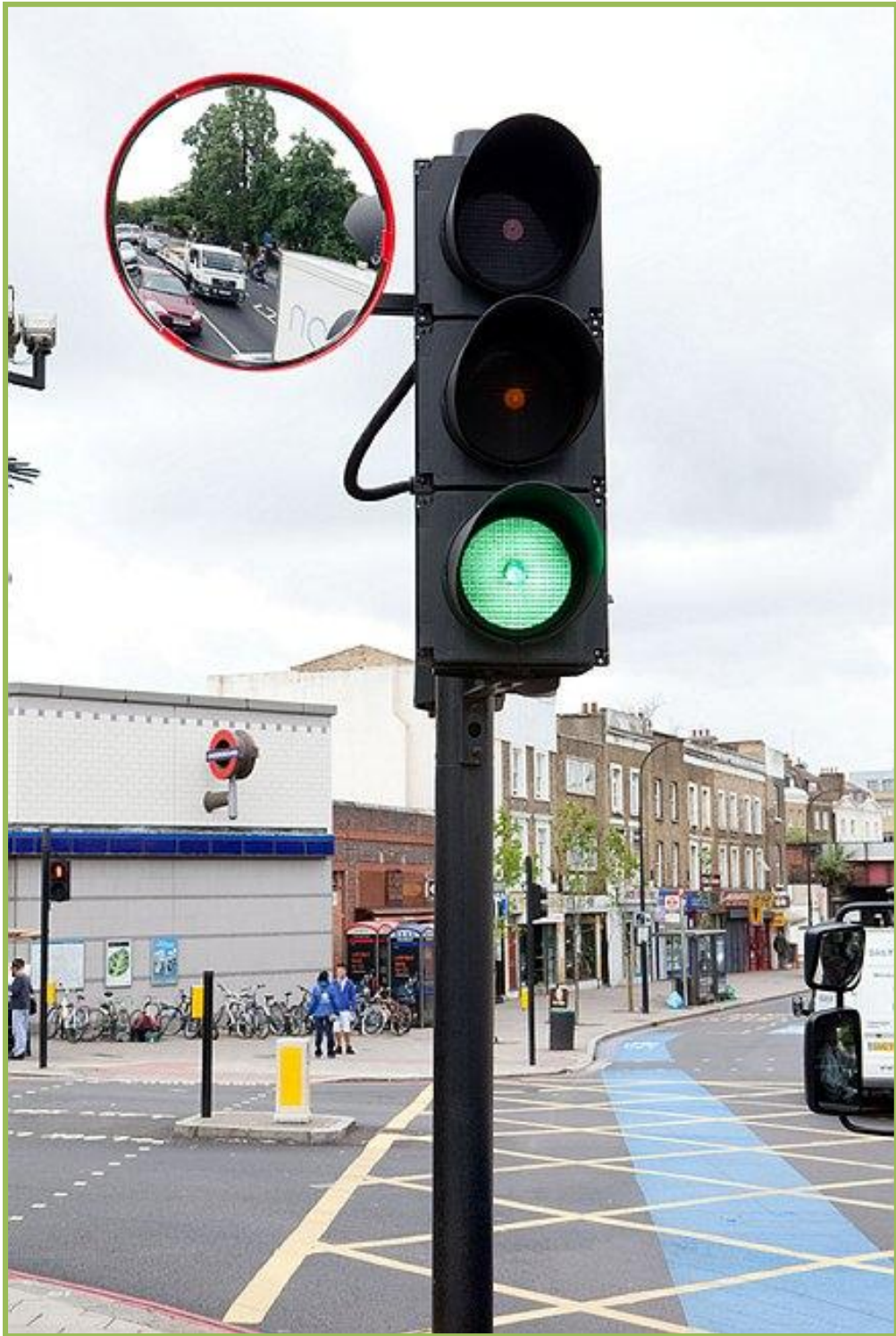
A blind spot safety trixi mirror on one of the superhighway pilot routes
