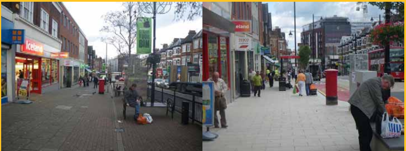
Before and after photos of Woodcote Road showing the re-laid footways, decluttering and general public realm improvements that have taken place as part of this Key Walking Route.
