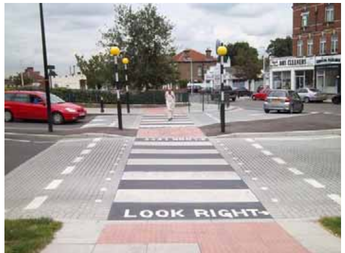
New zebra crossing outside South Woodford tube station to enhance access to the public transport network for those on foot and that supports a more permeable pedestrian environment in this popular location.
