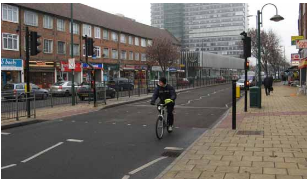
New signalised pedestrian crossing at Tolworth Broadway, Kingston. This new facility replaced a subway and the effects were monitored by TfL.
