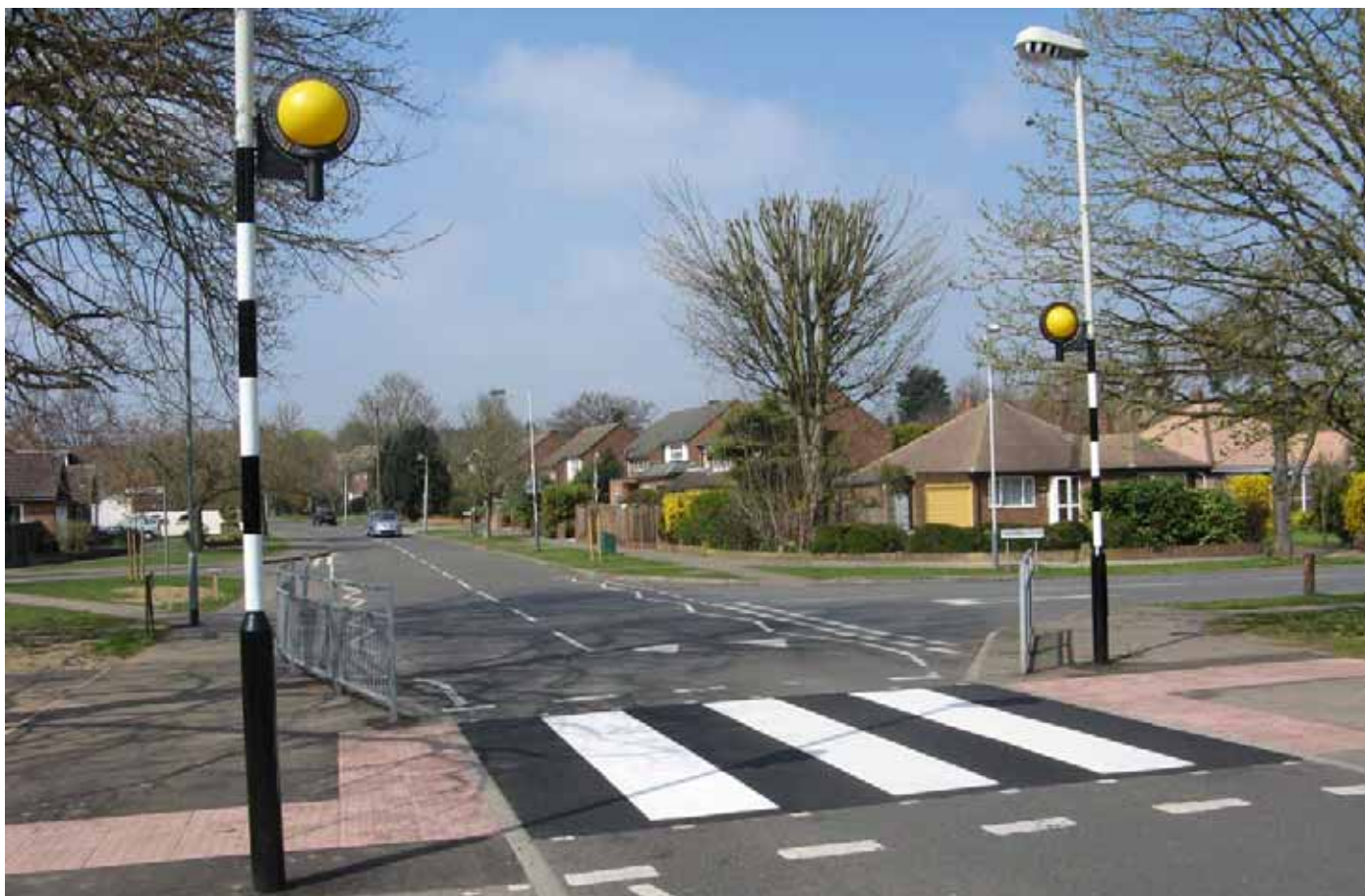
Swakeleys Drive zebra crossing, Hillingdon, using new 'Zebrite' technology to enhance visibility for pedestrians and motor vehicle drivers.
